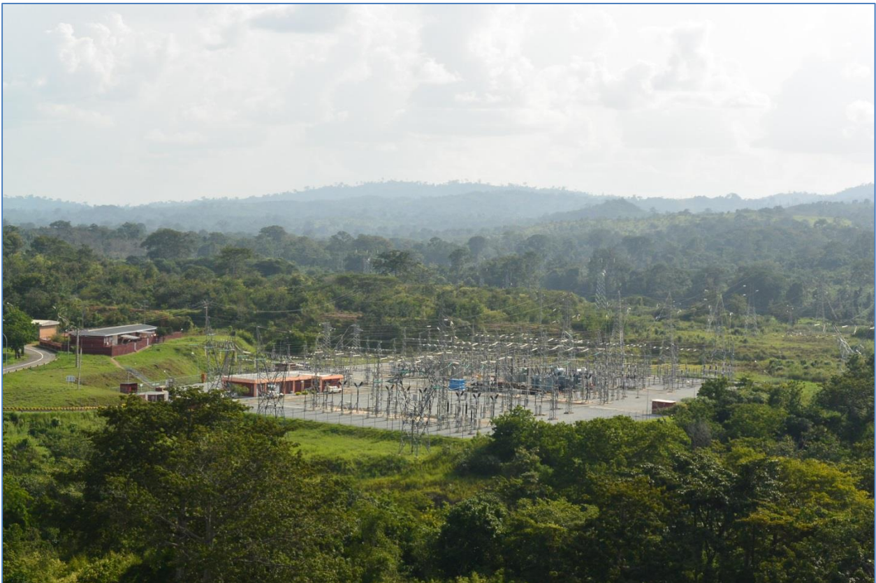
Figure 5-5 CIE Hydroelectric Power Station, Kossou
