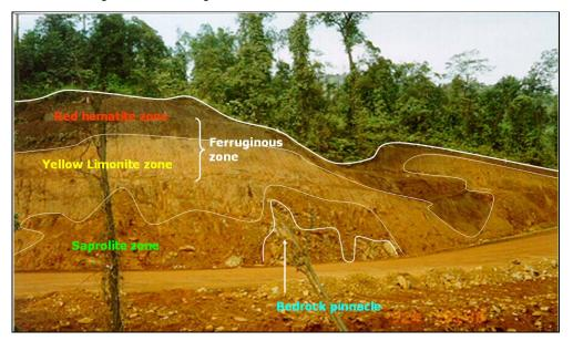
Figure 4-12: Geology Profile West Block (Photo PTI)
