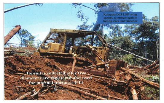
Figure 4-21: Topsoil Removal (Photo PTI)
