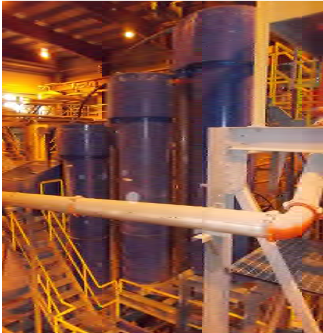
Figure 13.3 – Carbon-in-pulp reservoirs at the Kiena Complex
