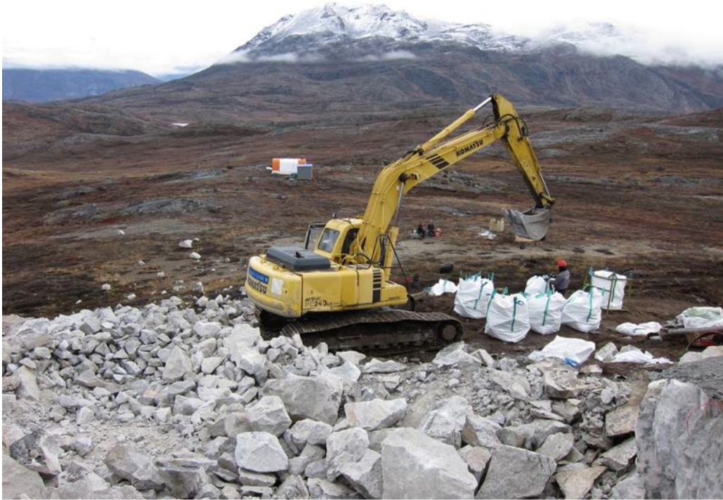
Figure 10-5 Blasted Material Ready for Loading: 2012 Bulk Sample
