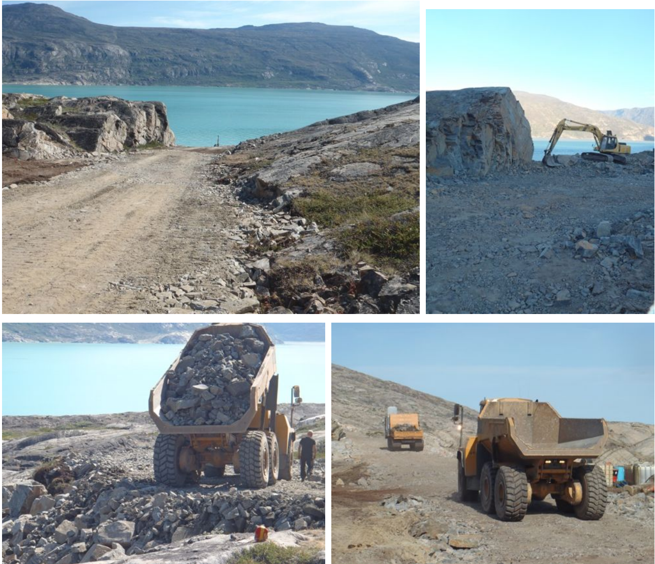
Figure 18-3 Road Construction in Progress
