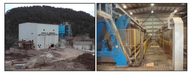
Figure 18-3 Aerial Filtration Circuit Building (left); Two Diemme Filter Presses (right)
