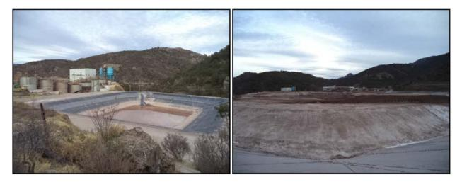
Figure 18-4 View of the new Rosario Tailings Water Pond with Capacity 10,000 m³ (on the left); View of the Dry Stack Tailings
