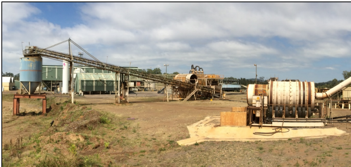
Figure 17.5: Feed preparation plant (scrubber in the foreground and trommel in the background)
