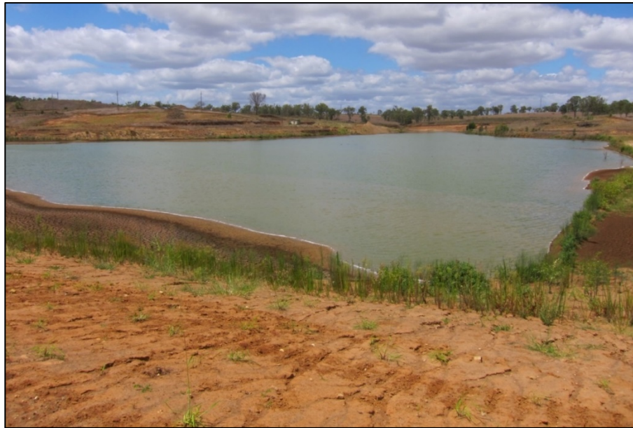
Figure 16.5: Goondicum tailings dam
