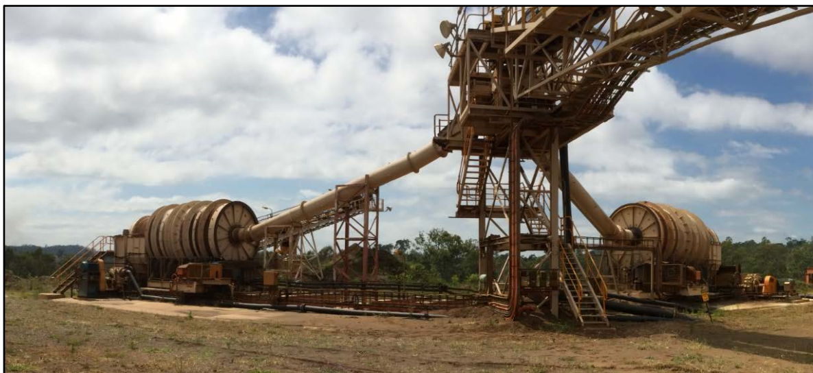
Figure 17.4: Feed preparation area dual scrubbing units
