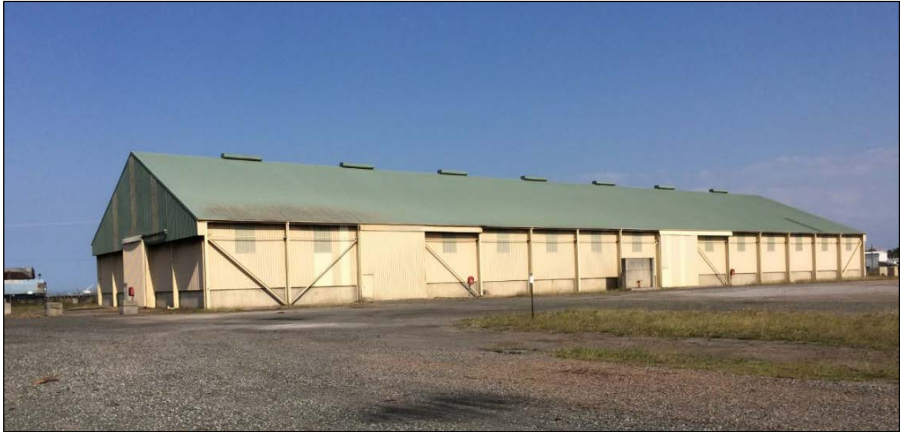
Figure 18.6: Ilmenite storage shed at the port
