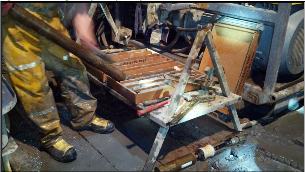
Figure 10-3 Placing Core (January 2013)
