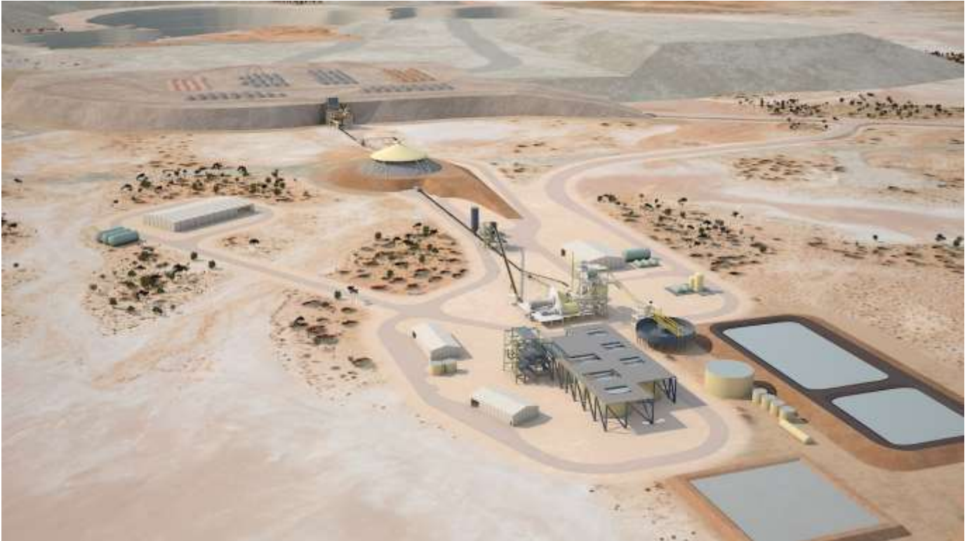
Figure 14: 3D image showing the layout of the planned 2.5Mtpa process plant with the Jupiter open pit in the background. The ROM pad lies between the open pit and the process plant.
