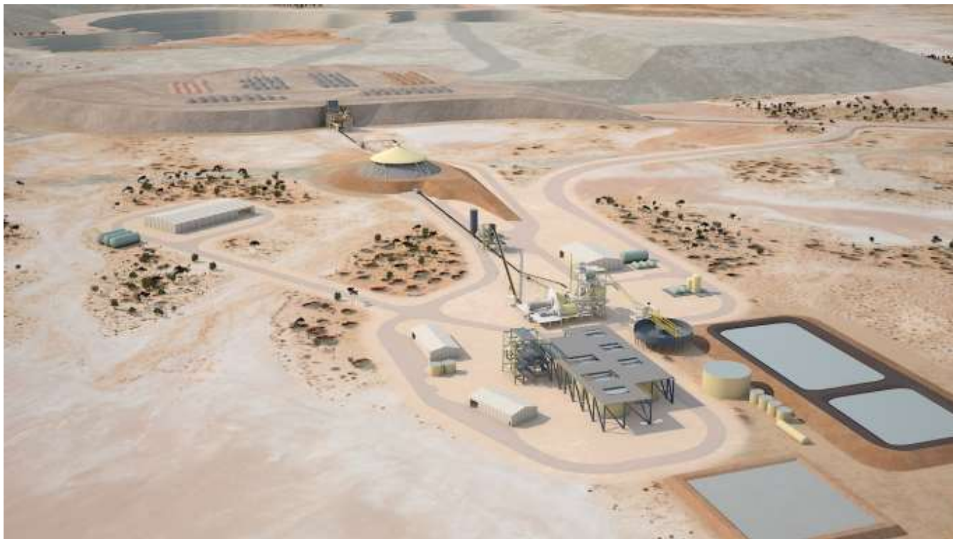
Figure E3 – 3D-image of new 2.5Mtpa CIL treatment facility with Jupiter open pit in the background.
