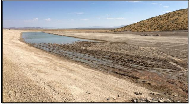
The RIBs should be located and designed to infiltrate water into the alluvial sediments of the Reese River Valley and located in a manner that will minimize re-circulation to the Cove Pit lake. Infiltration of dewatering water to a series of Rapid Infiltration Basins has been used at the McCoy Cove site in the past to re-introduce dewatering discharge into the groundwater system.
