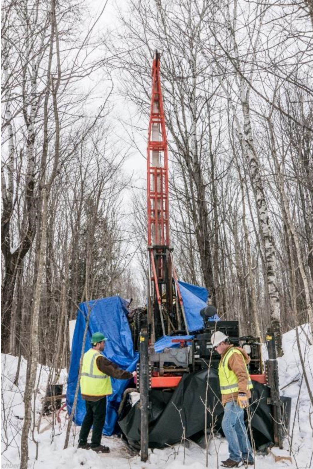
Figure 10.2: Winter Drilling at the Section 5 Area
