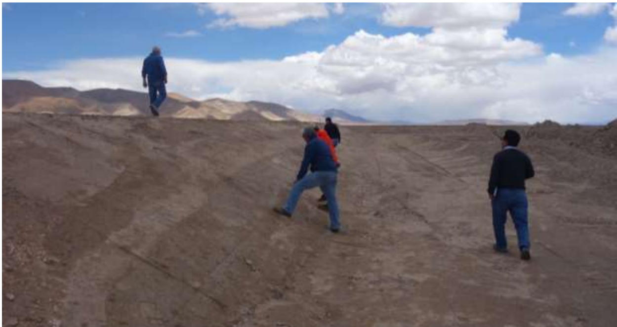
Figure 17.3 Testing of Berm Material
