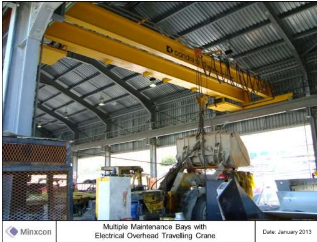
Figure 68: Multiple Bays with EOT Crane
