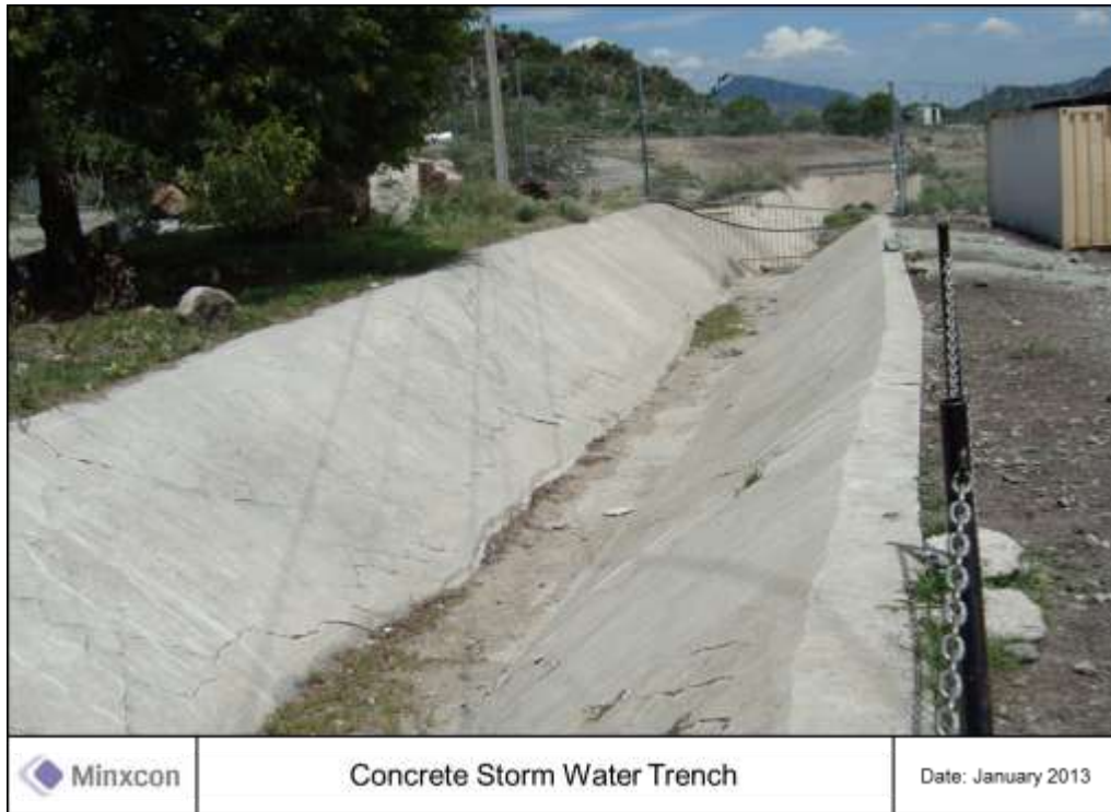
Figure 58: Trench for Storm Water Control
