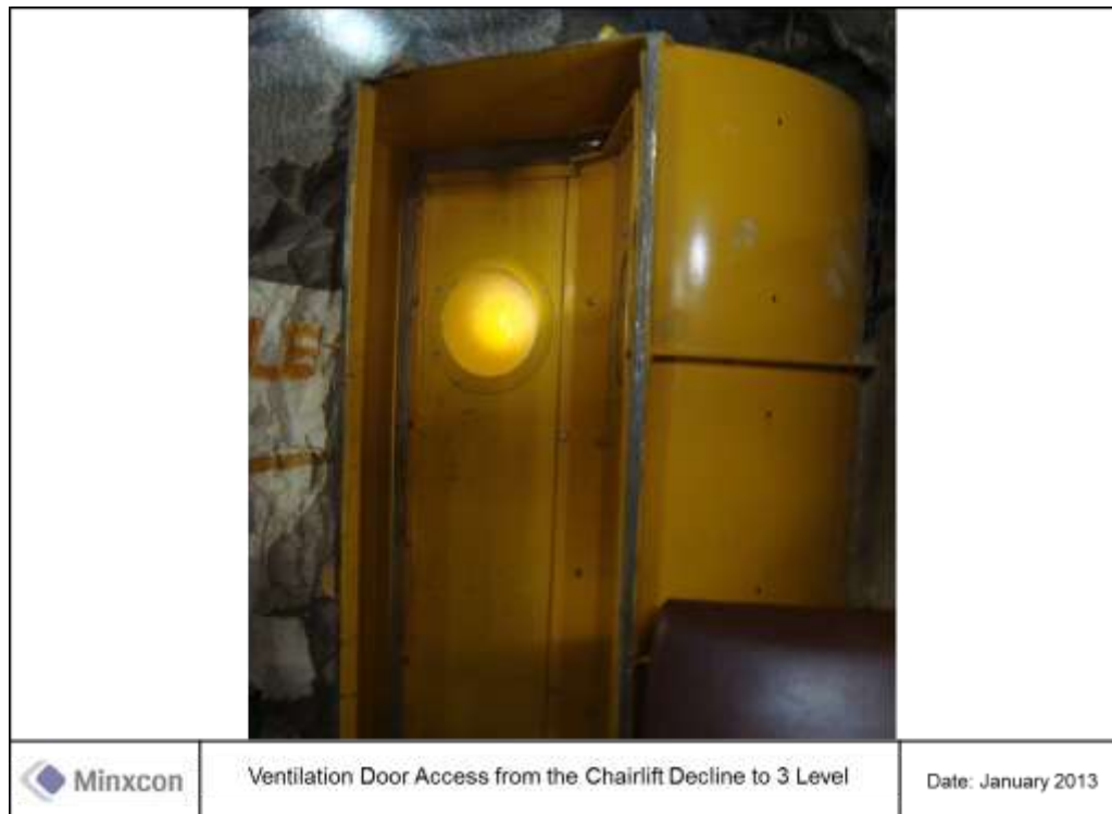
Figure 69: Ventilation Door and Access from Chairlift Decline to 3 Level
