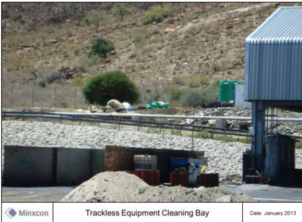
Figure 57: Cleaning Bay for Trackless Equipment
