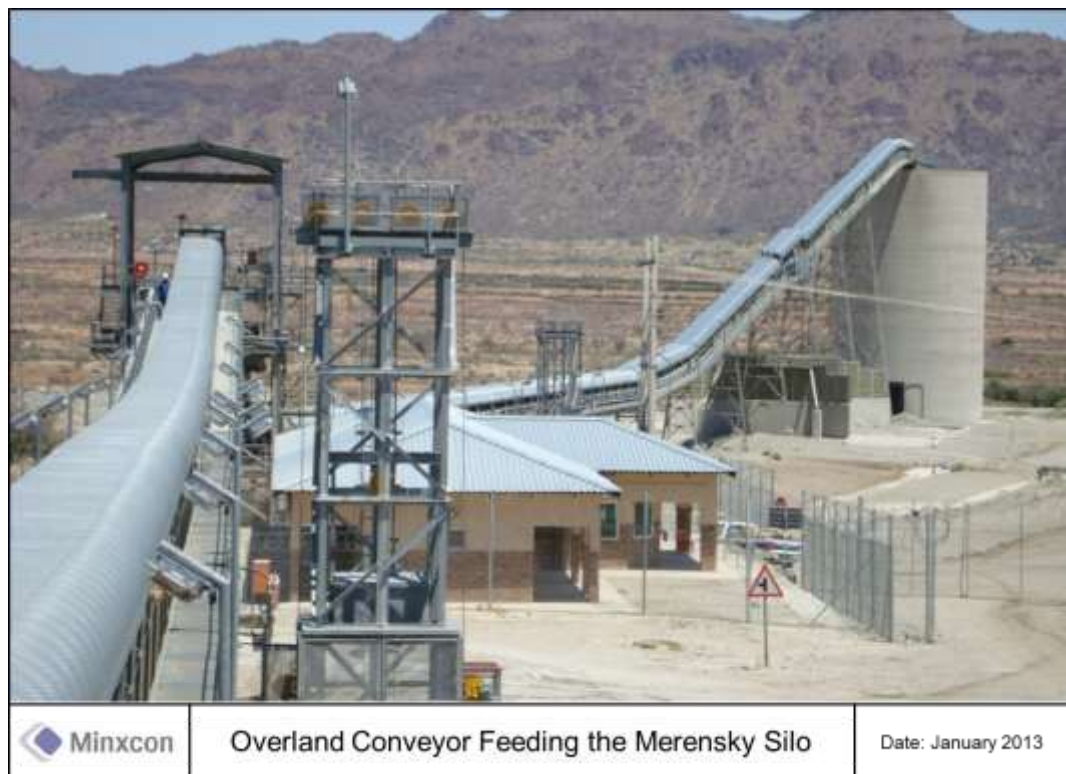
Figure 60: Overland Conveyor Feeding the 3,000 Tonne Merensky Silo
