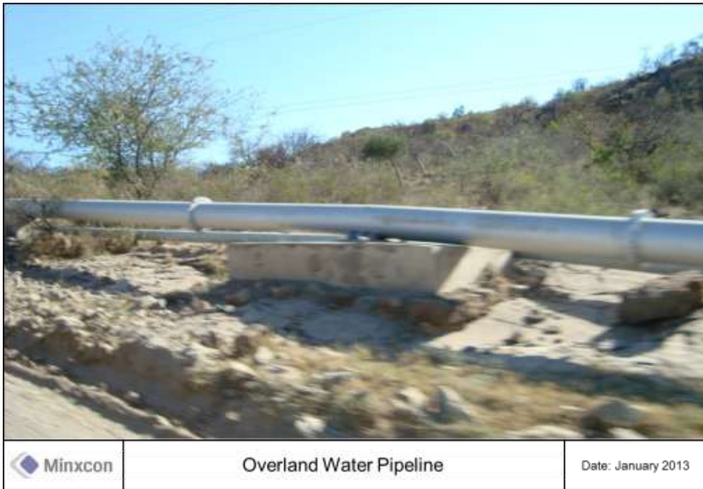
Figure 56: Overland Water Supply Pipeline
