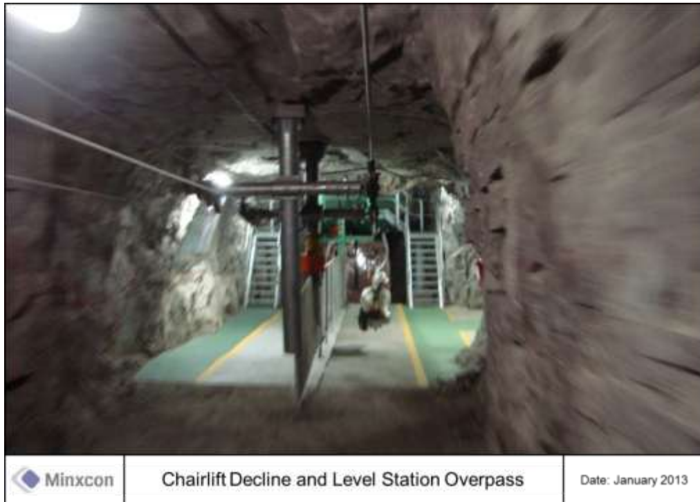
Figure 63: Chairlift Decline and Level Station Overpass
