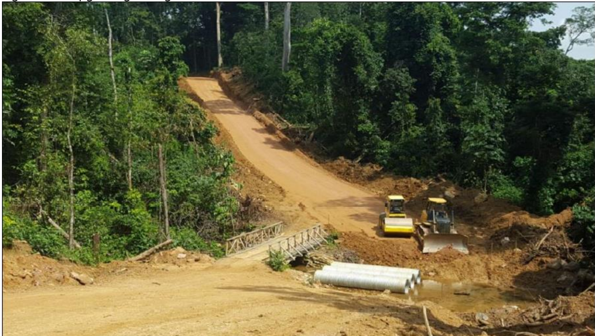
Figure 13.1 Upgrading of Logu-Bisie Access Route
