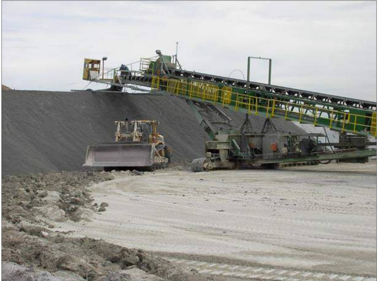
Figure 17-9 Stacker and Dozer Ripping the compacted surface
