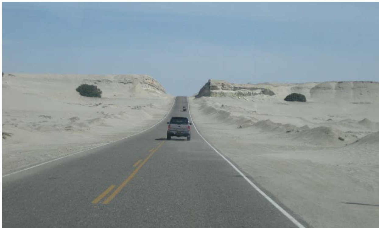
Figure 5-7: Chiclayo-Bayovar Road on the Bayovar 12 Concession with the Tablazo in the Background
